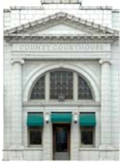
MI53004... 1/16 COURTHOUSE FRONT
